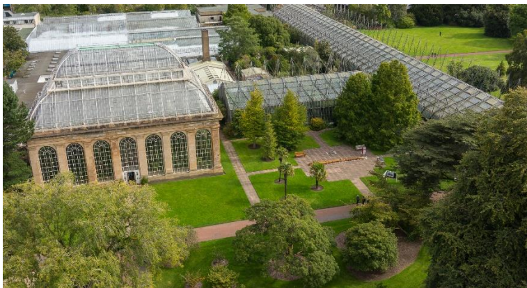
A drone photo that shows the existing public and research houses but also the decrepit boiler house to be replaced by the shiny new efficient energy centre.
