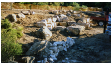
The team has constructed rock walls, paths, and steps in the Gardens.
