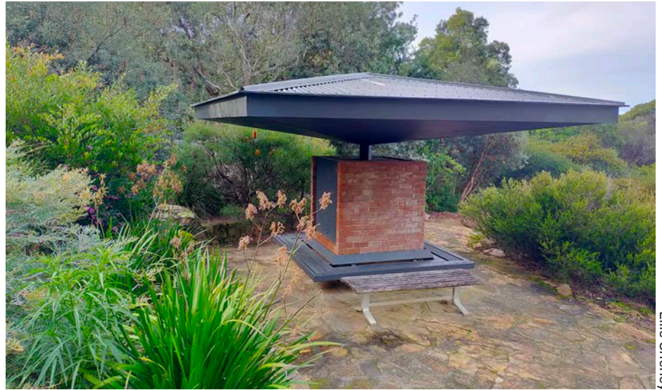
Refurbished Otto Ruzicka shelter in Section 37, north of the Rainforest Gully.
